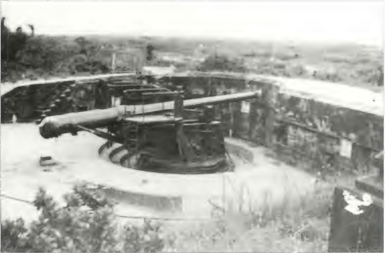
Figure 5.77. Battery Gunnison, circa 1941 prior to converting the battery to barbette mounted guns. Note the predominance of herbaceous vegetation at this time. Also note the weathered black paint on the concrete surfaces (GATE 7834).
